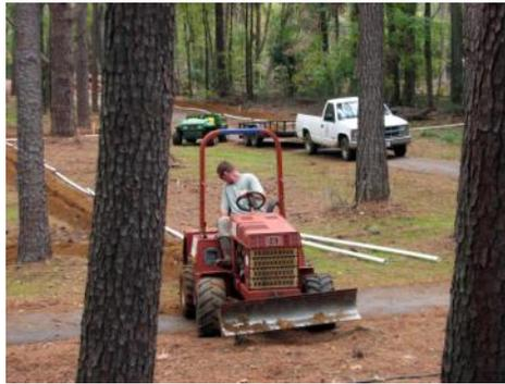
*Brad Waguespack operates a ditch witch in the SFA Rec Trails and Gardens to create irrigation lines.*
